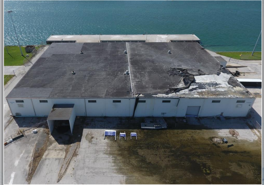
Post Hurricane Matthew: Northside Warehouse Roof Damage
