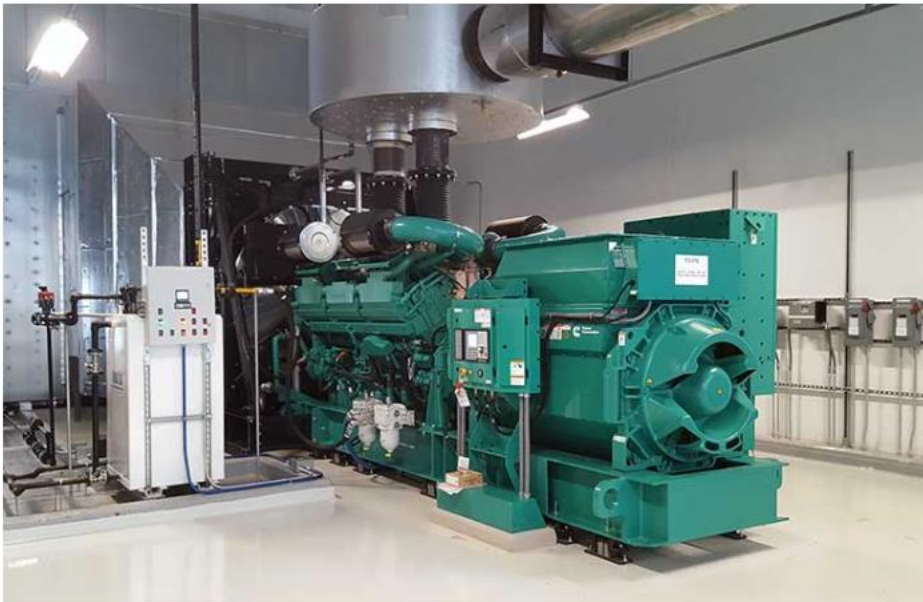
One of the 28 Cummins 2750kV backup generators at the CloudHQ Manassas Corporate Center 1 data center. (Photo: Rich Miller)
