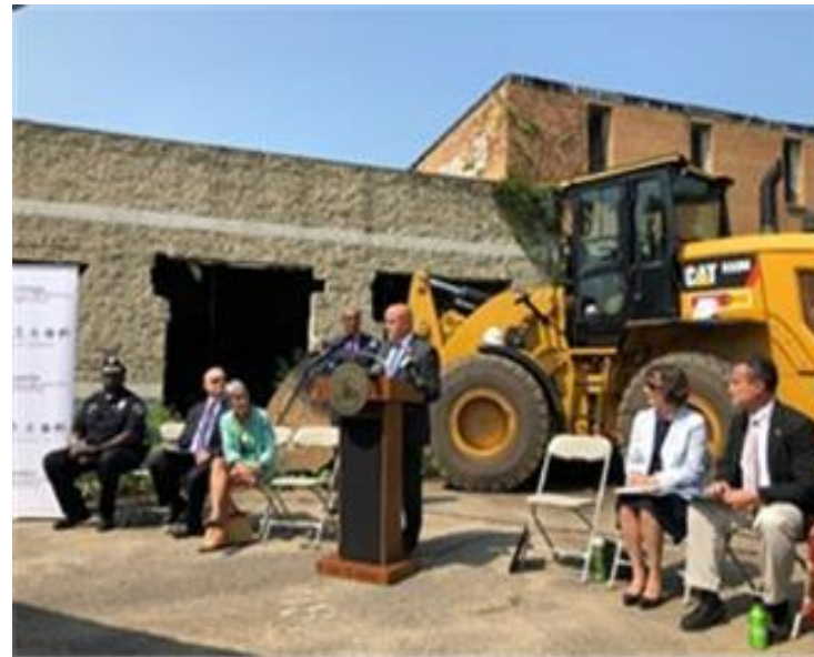
AWP Site Demolition/Press Event Camden, NJ
