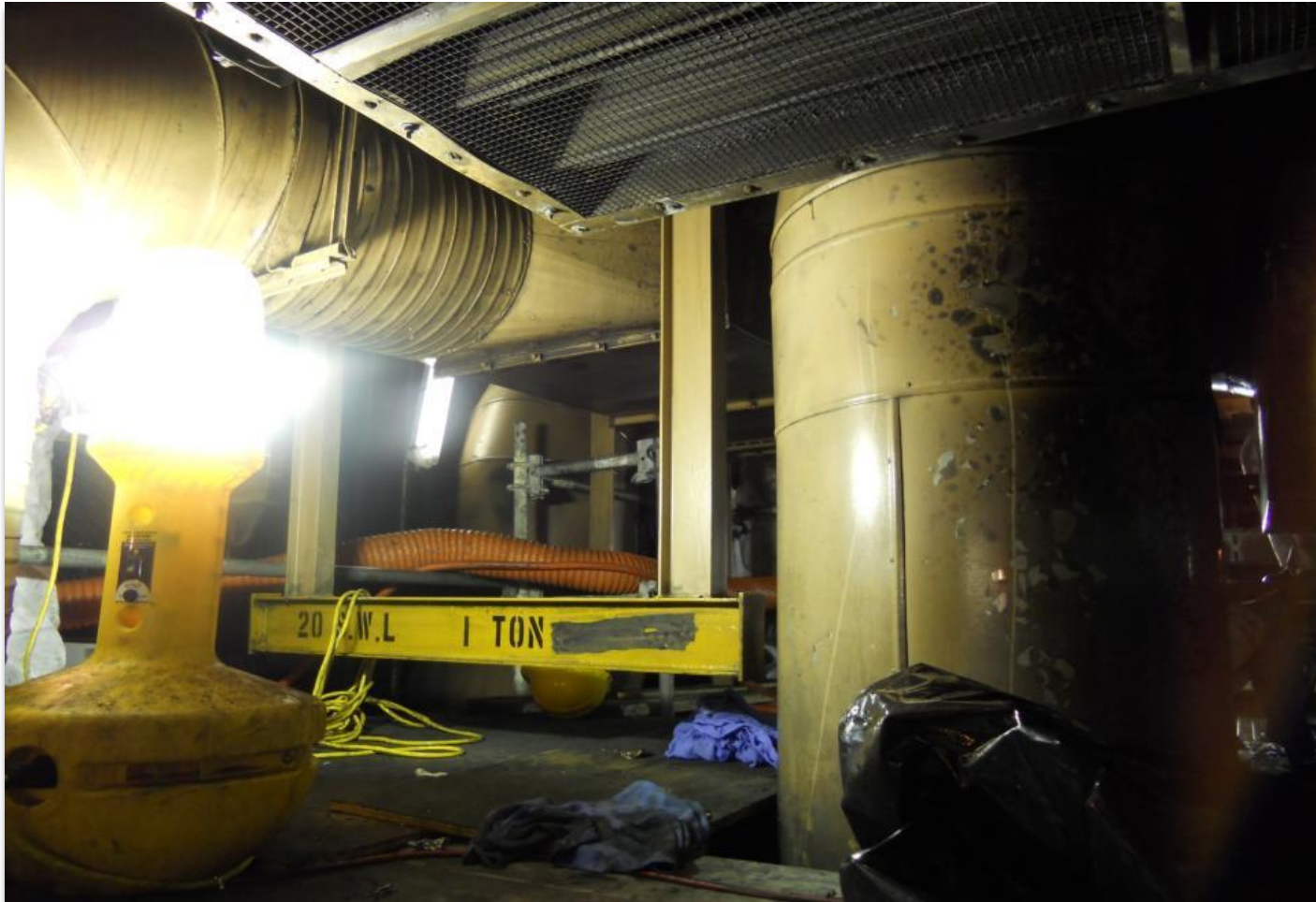
Generators On The Pier Supplied Power
