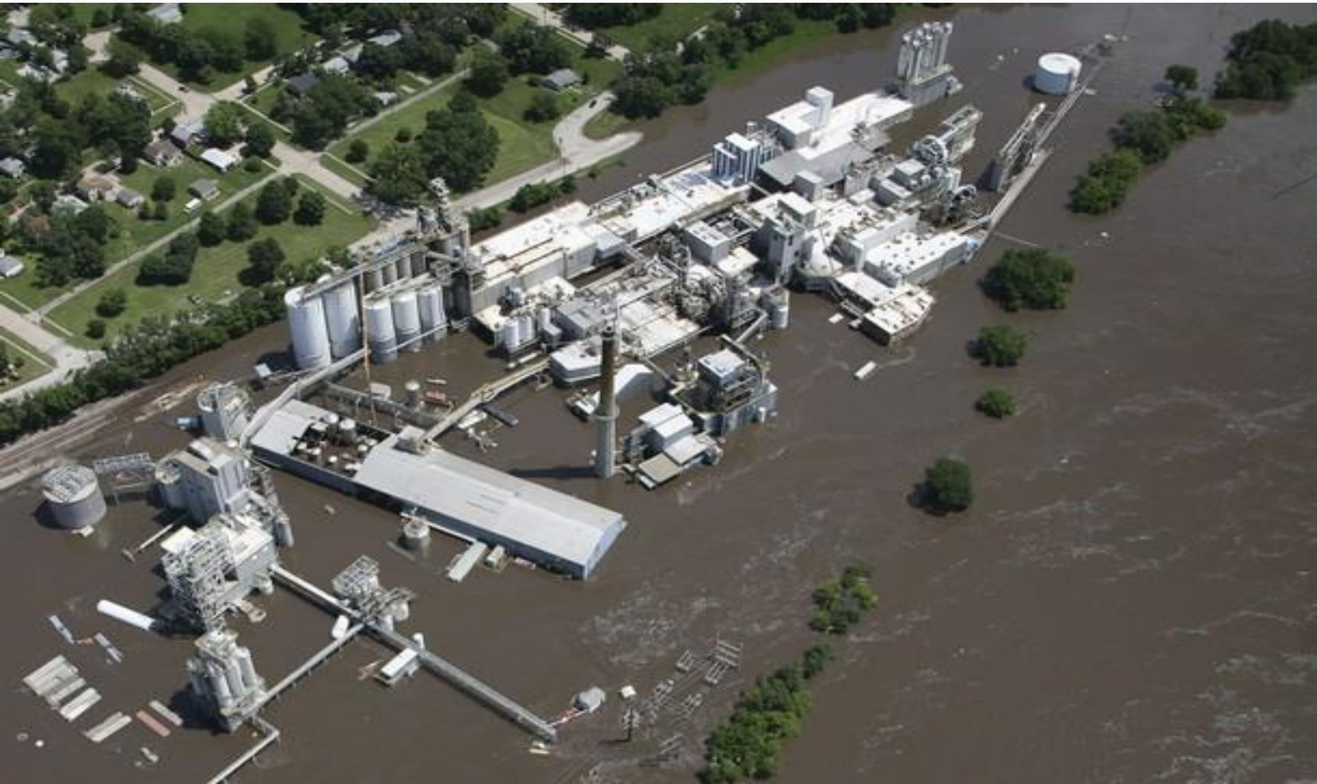
VIEW OF FLOODED PLANT, FRIDAY, JUNE 13, 2008
