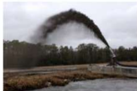
TLP of dredged material at Pepper Creek Delaware
