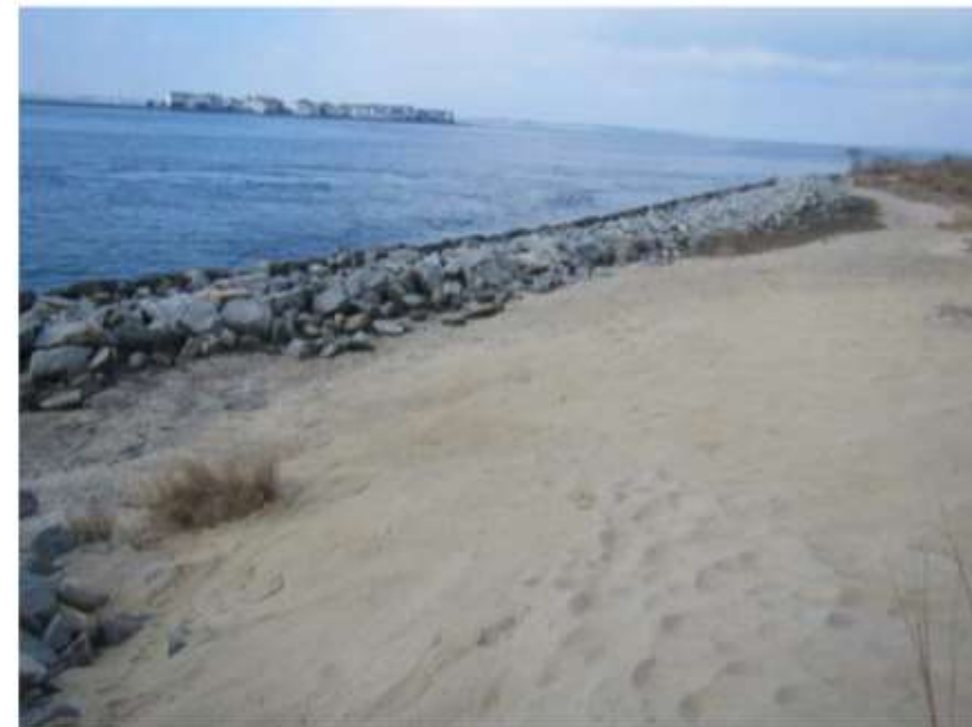
Revetments along Bubblegum Beach, Rehoboth Beach, DE.
