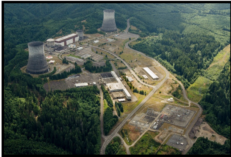
The Satsop Business Park as seen today. The two iconic cooling towers can be seen from miles away.
