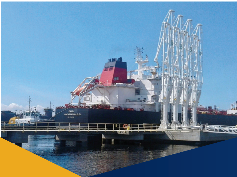
A petroleum vessel offloads fuel at Port Tampa Bay on September 7, 2017
