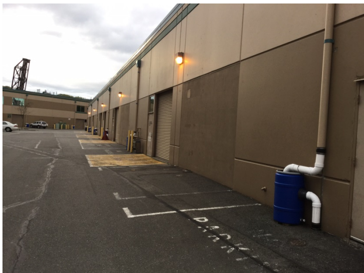
Figure A-2 - Barrels installed onsite
