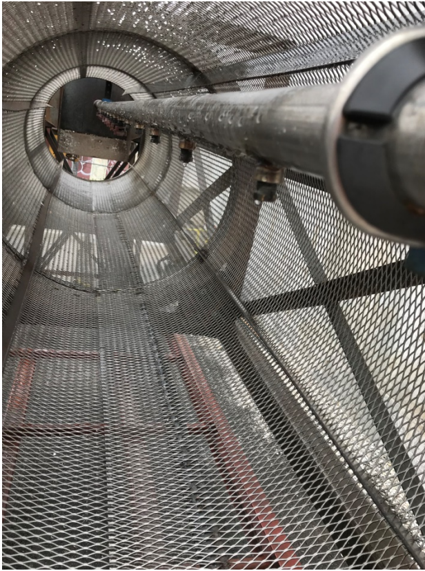
Figure B-1 - Fixed Water Pipe
