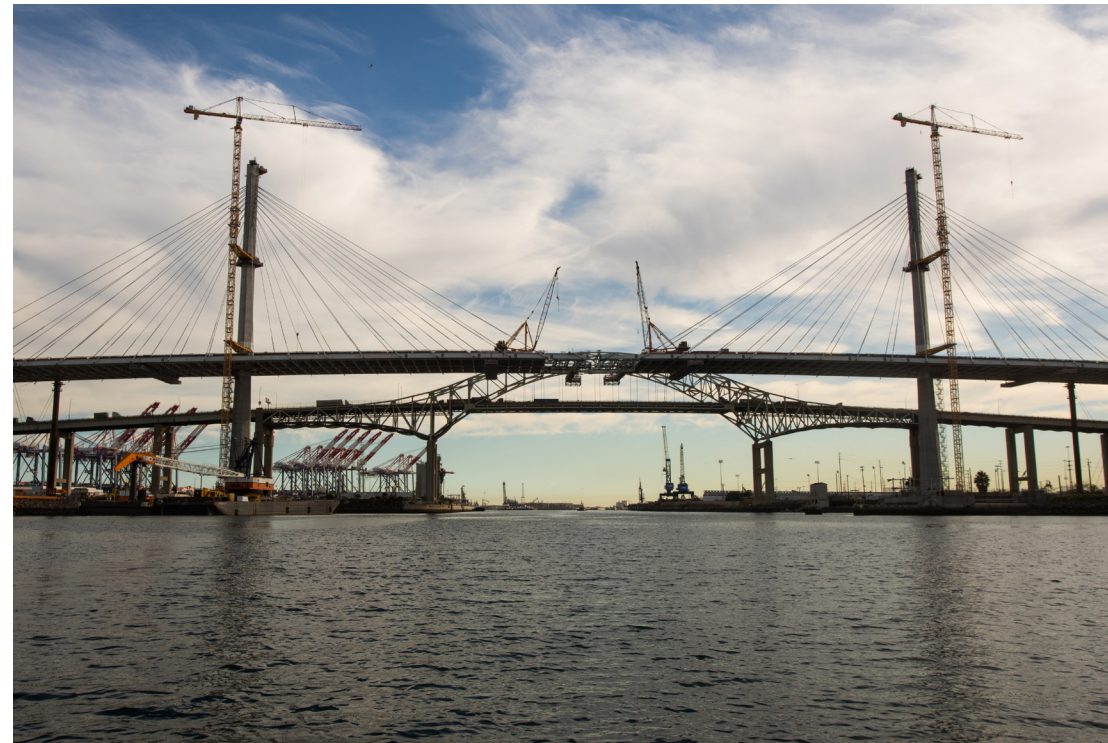
New bridge nearing completion, with Gerald Desmond Bridge in the background
