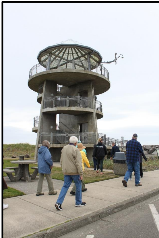
Tour guests make their way up the Centennial Viewing Tower for a look at the Grays Harbor Navigation Channel and other Corps infrastructure.
