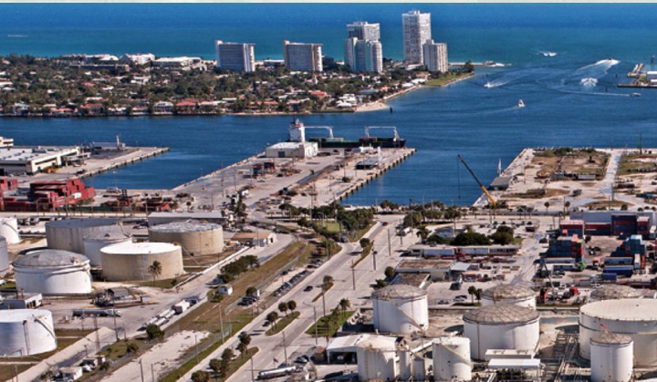
Warehouses, Storage Yards, Storage Tanks
