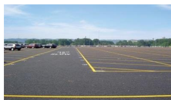
Completed Terminal 6 auto storage yard at Port of Portland with porous pavement
