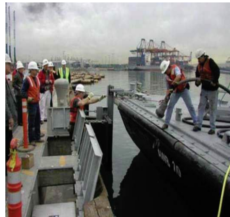
On-shore power installation
