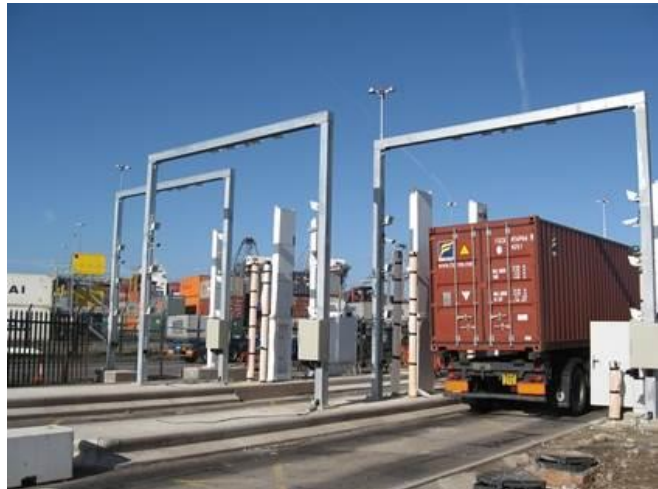
Port of Southampton UK: Three OCR Gate systems integrated into radiation portals for US Customs.
