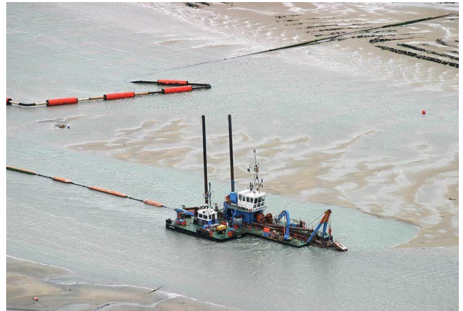
Dredging at Port of Honfleur, France
