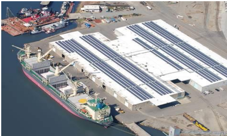
Port of West Sacramento solar roofs
