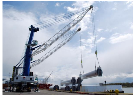
Off-loading of wind turbine components at the Port of Vancouver, USA
