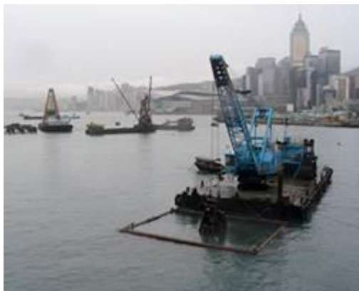
Turbidity curtain deployment during dredging at Port of Hong Kong
