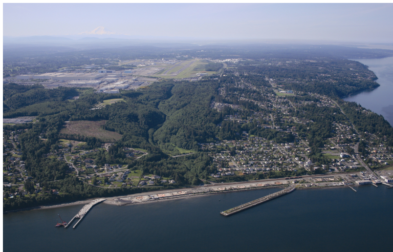
Figure 7: Aerial of finished park and beach.
