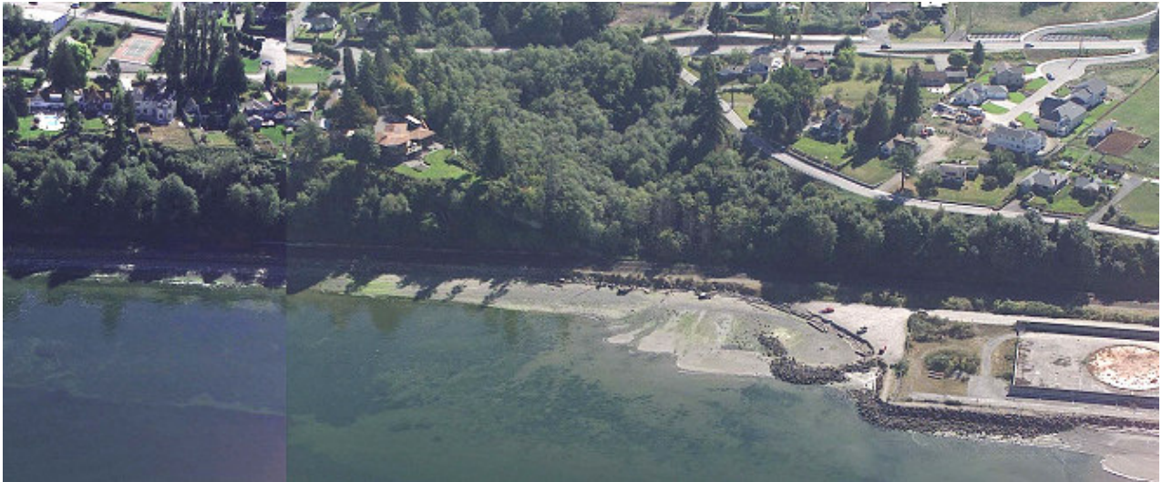
Figure 3: Pre-construction photo on eastern side of proposed enhancement looking west toward abandoned tank farm.
