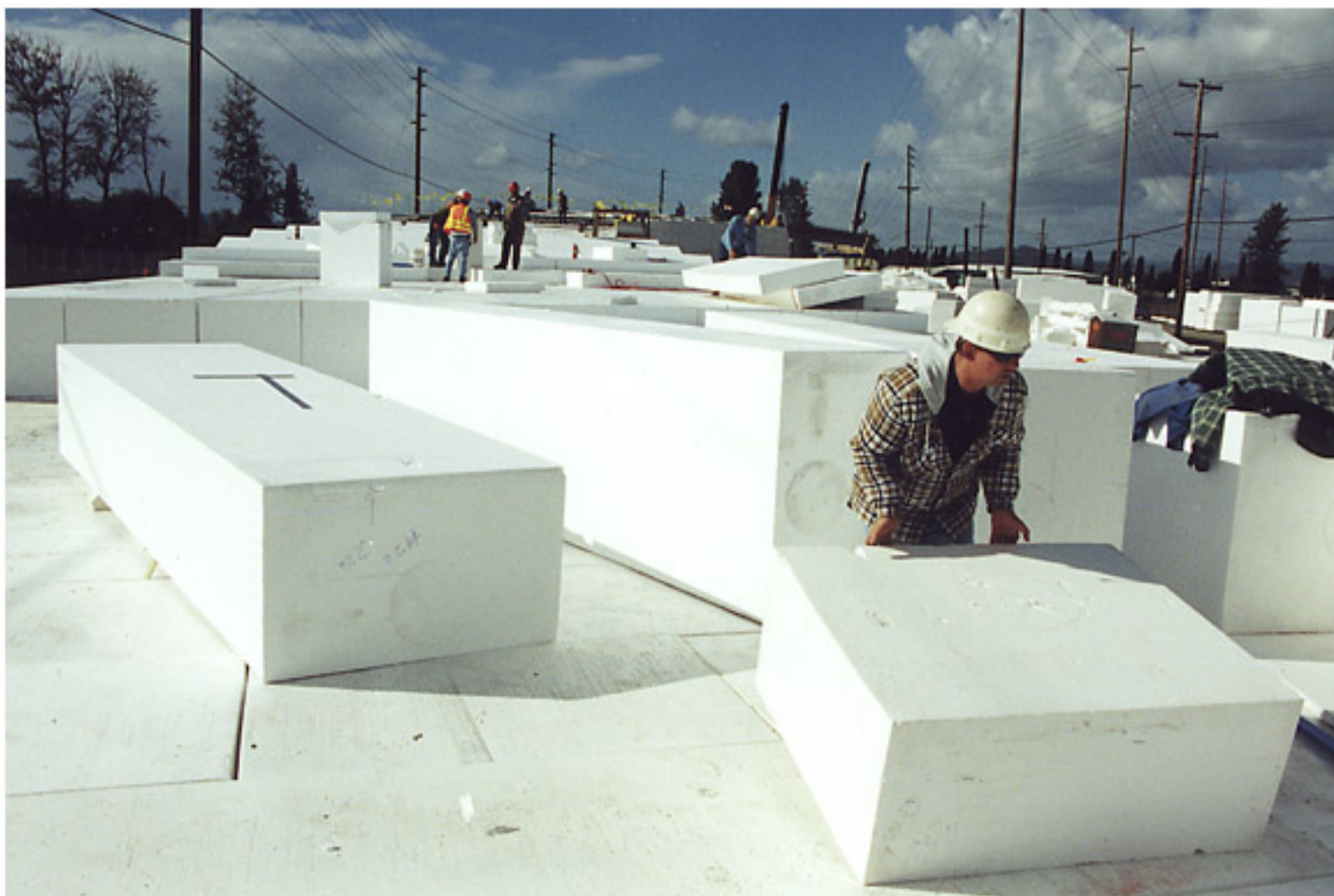
An Ostrander Rock and Construction worker moves Geofoam blocks into place. Each 16 foot-long block weighs approximately 280 pounds.
