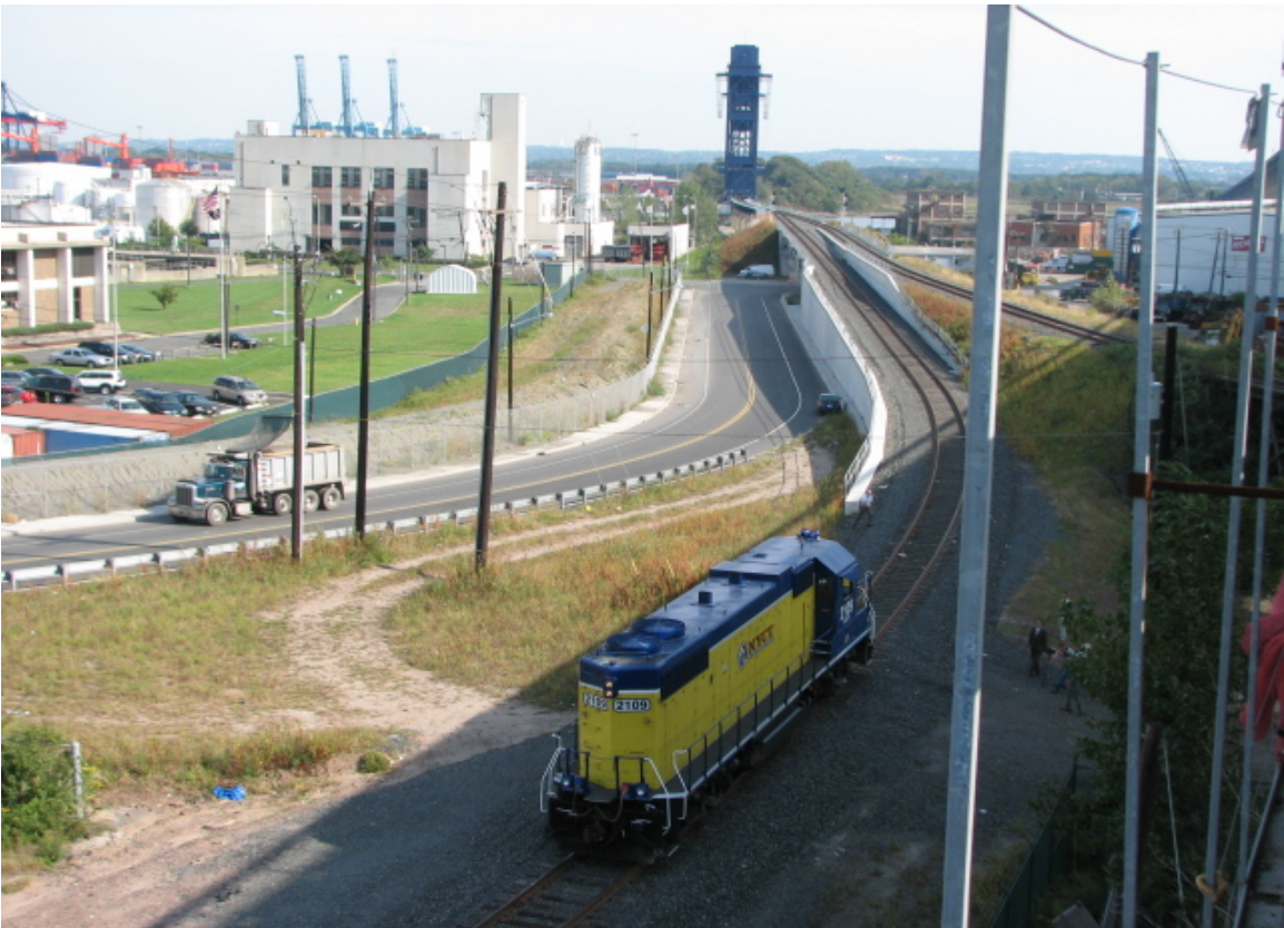
Photo 14: Chemical Coast Connector to the AK Bridge.
