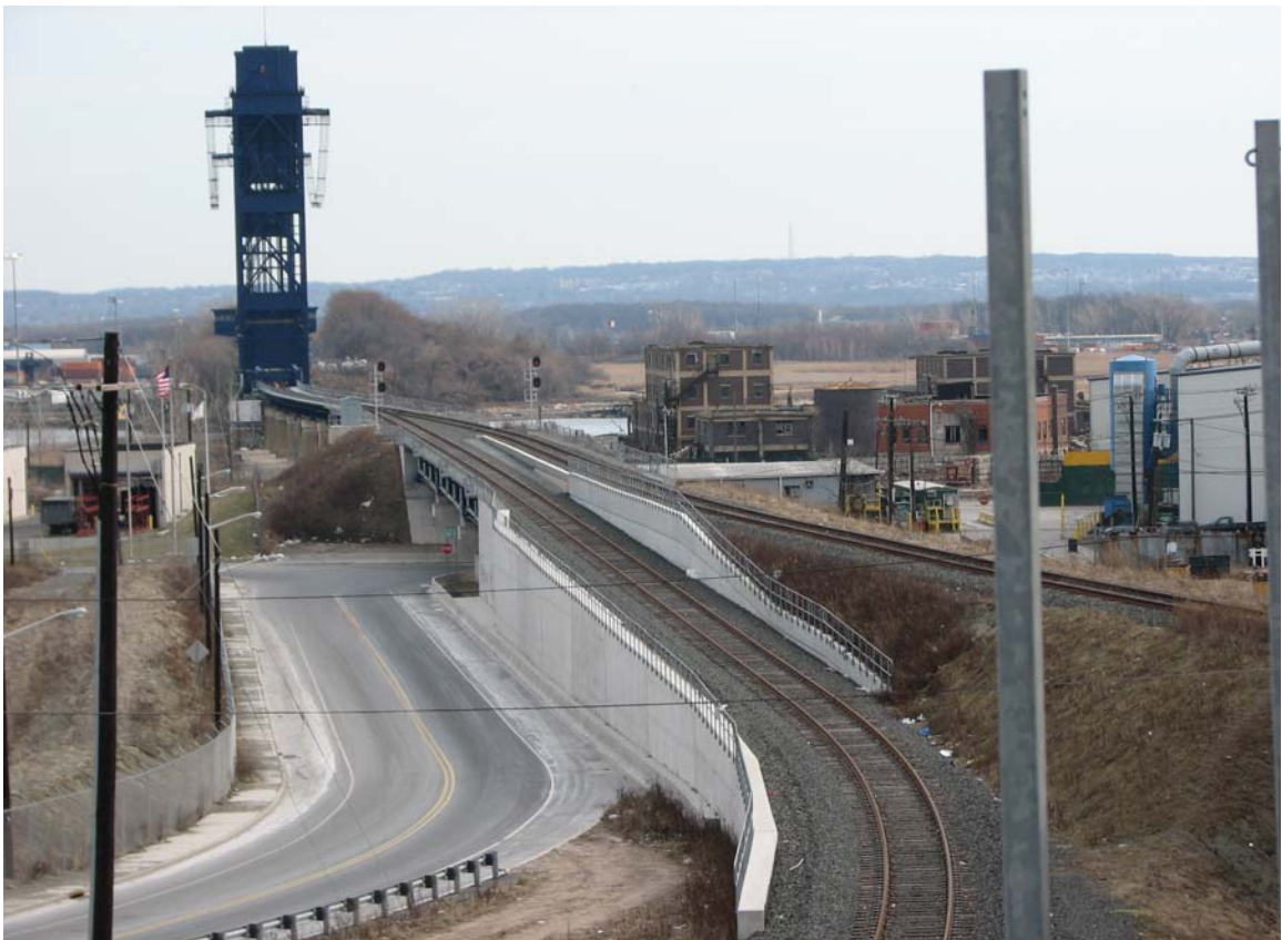
Photo 8: Completed Elevated Connector and Realigned Bayway Avenue.
