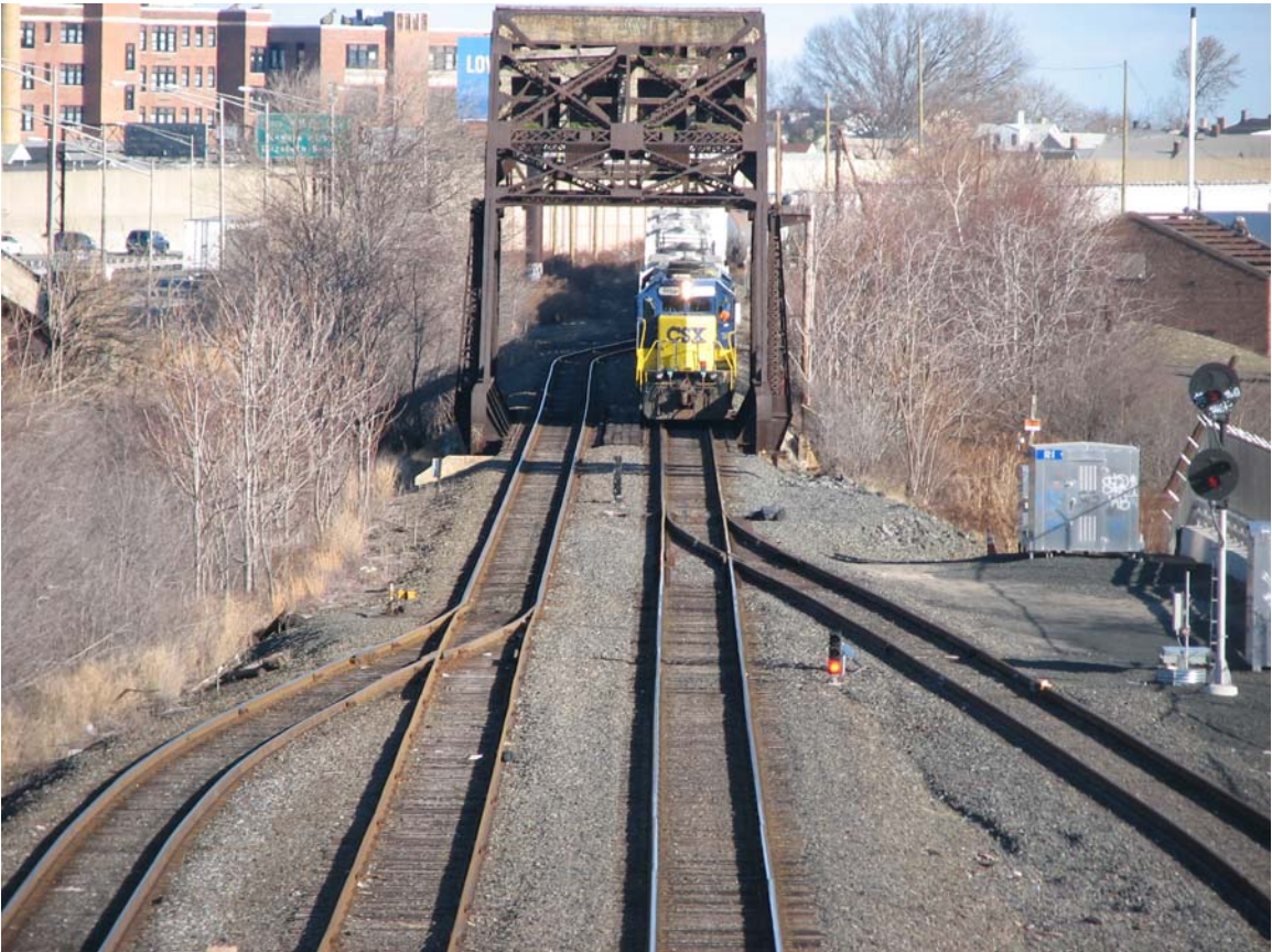
Photo 12: Connection to the Conrail Chemical Coast Line.
