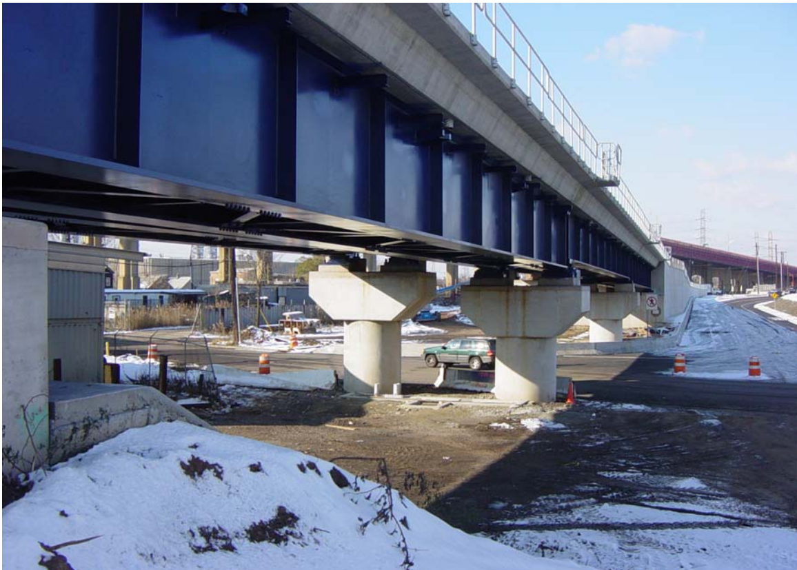
Photo 6: Completed Three Spans of Twin Bridge at Amboy Avenue.
