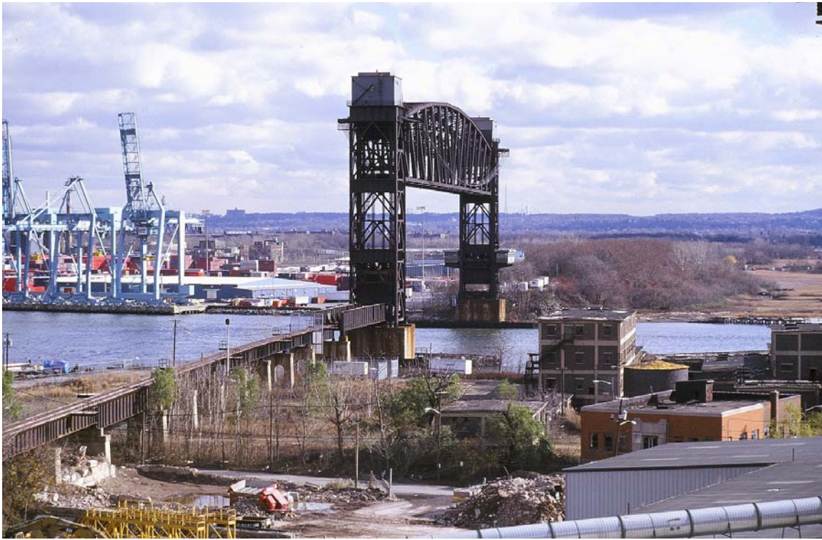
Photo 1: Deactivated Staten Island Railroad / AK Lift Bridge
