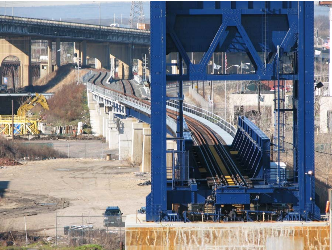
Photo 11: Chemical Coast Connector to the AK Bridge.
