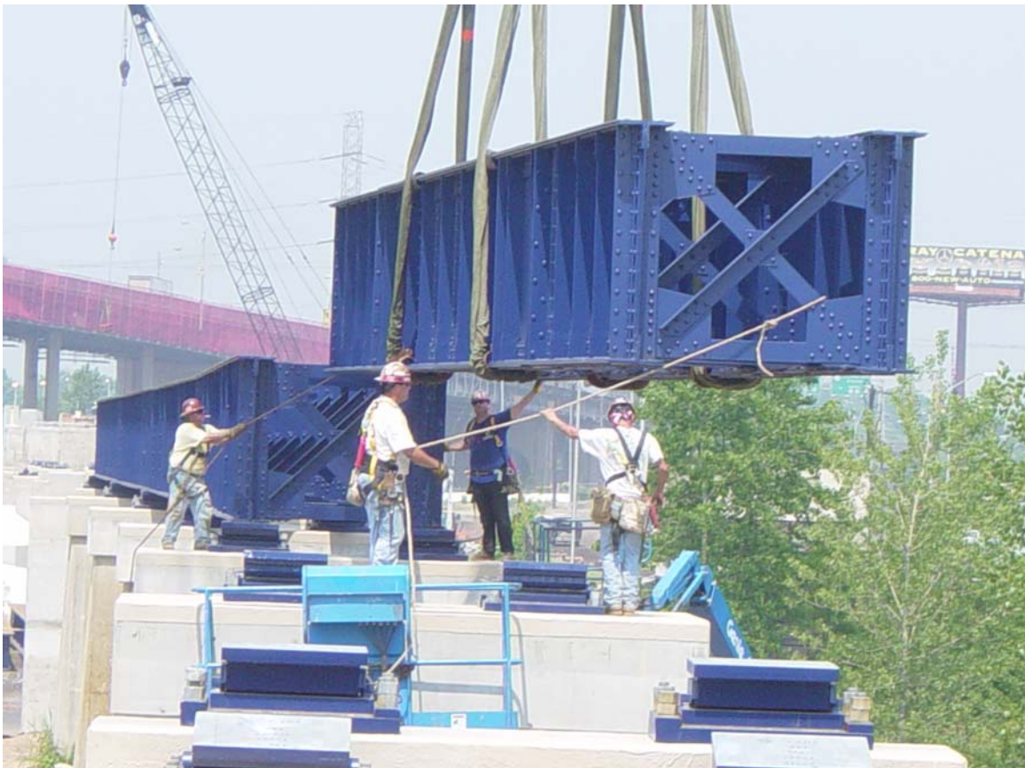
Photo 4: Reinstallation of the Rehabilitated Approach Spans.
