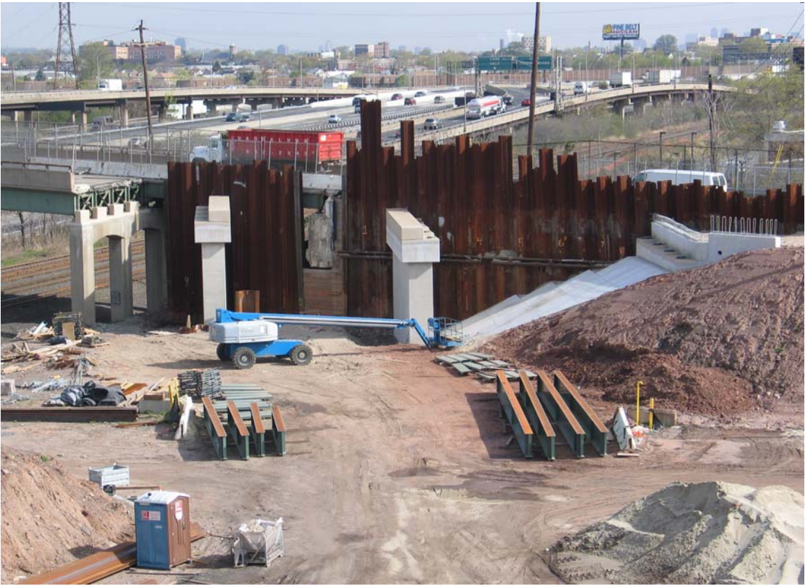
Photo 9: Bayway Avenue Bridge Reconfigured to Accommodate New Track.
