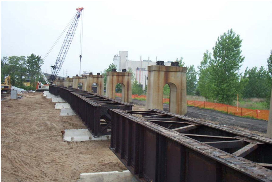
Photo 2: Removal of SIRR / AK Bridge Approach Spans for Rehabilitation.
