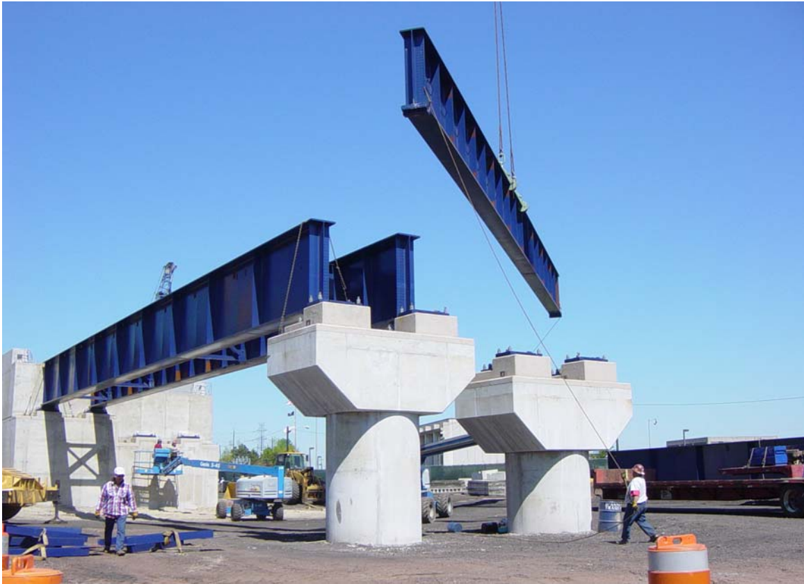
Photo 5: Installation of New Bridge at Amboy Avenue.
