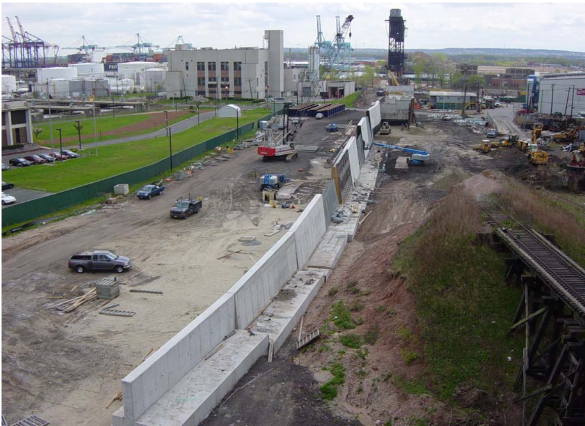
Photo 7: Construction of the New Connector Retaining Structure.
