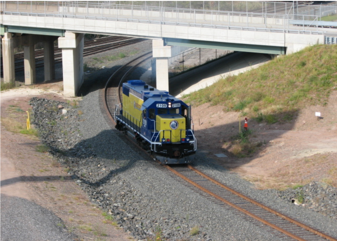
Photo 13: Connector Under the Bayway Avenue Bridge.
