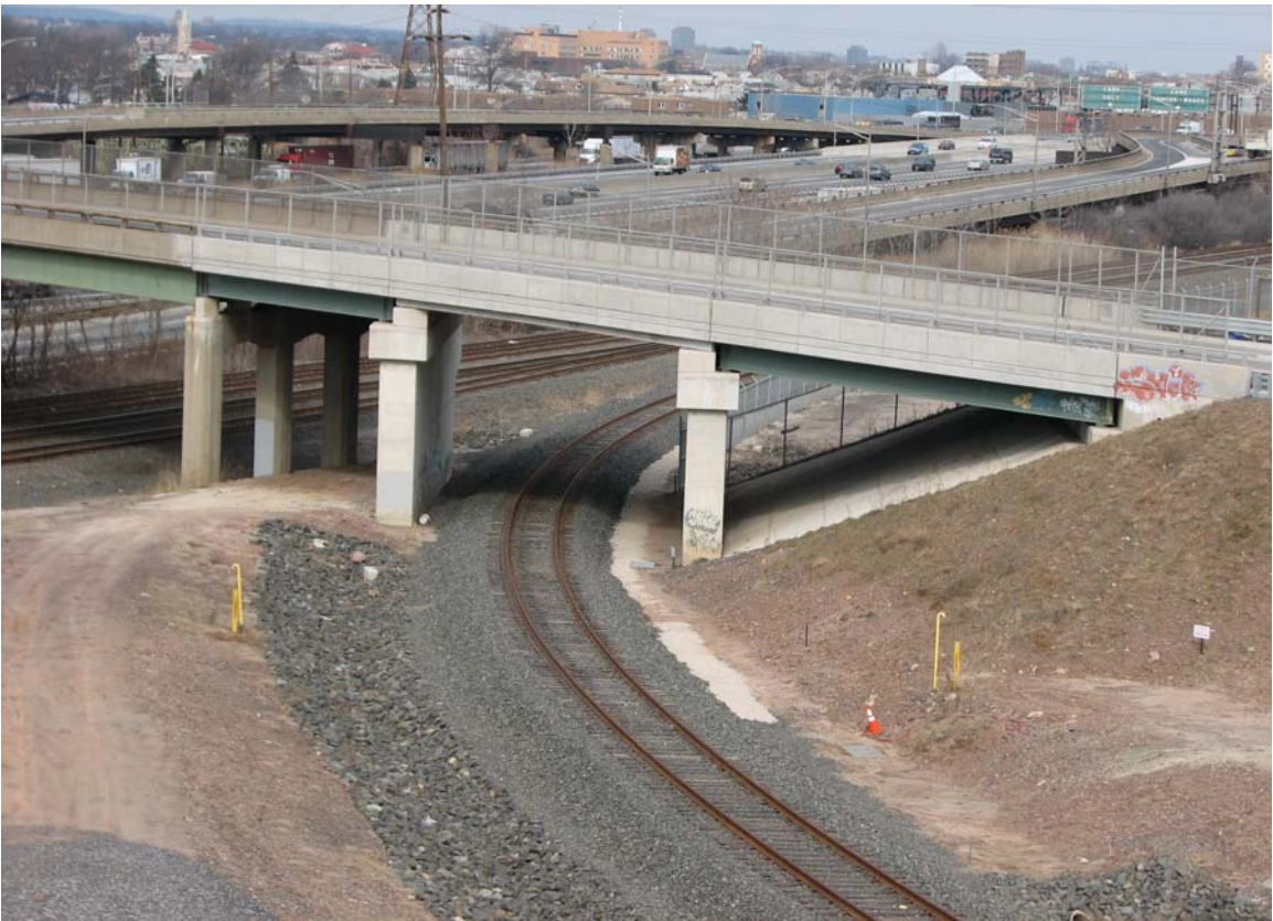
Photo 10: Bayway Avenue Bridge over the New Connector Track.
