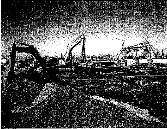
The sequencing of sump excavation required overburden to be removed for reuse on site, followed by excavation of the sump material for transport off site.
