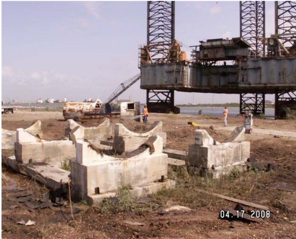
Quintana Marine site with ZEUS MODU and associated abandoned tank
