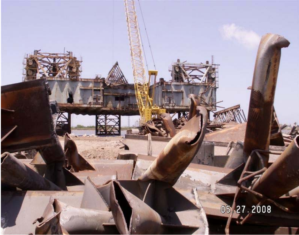
ZEUS MODU demolition
