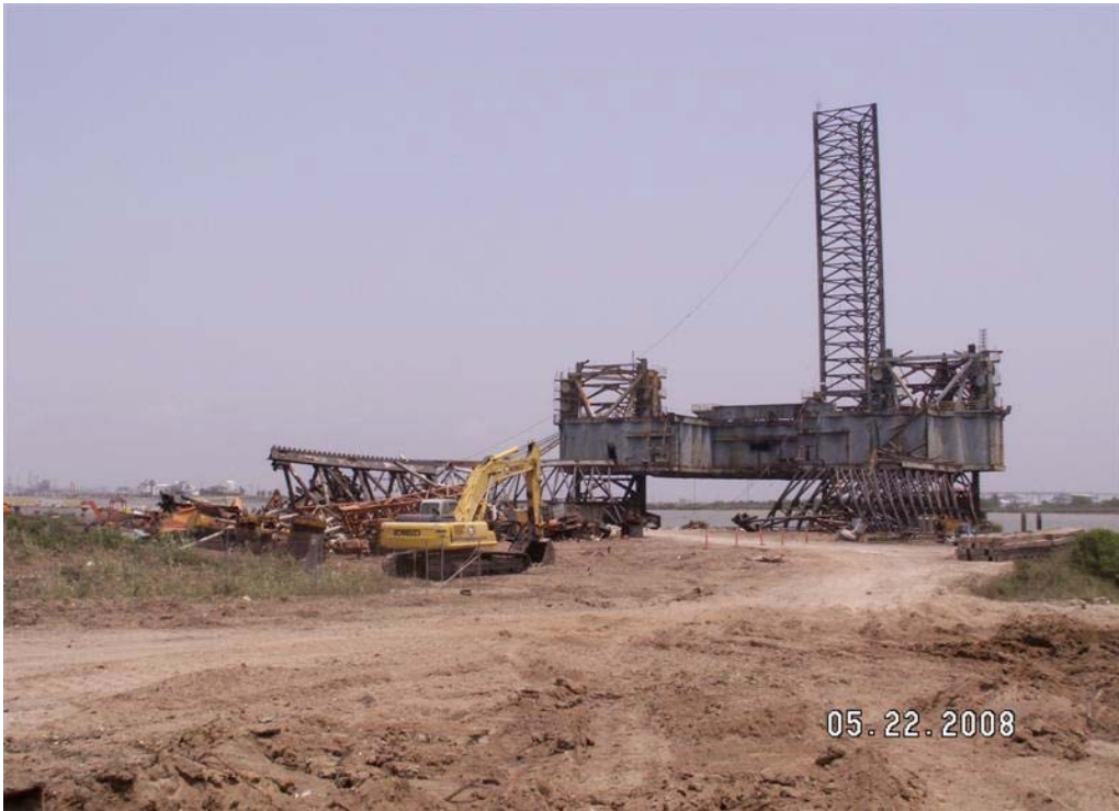
ZEUS MODU demolition
