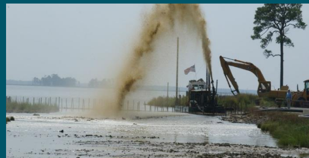
Thin layer capping over marsh
