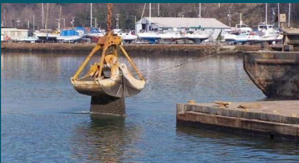
Thin layer placement with rehandling bucket
