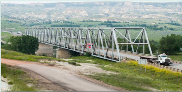
Photos courtesy of: North Dakota DOT (left); Cal Klewin, Executive Director of the Theodore Roosevelt Expressway Association (right); North Dakota DOT (bottom).
