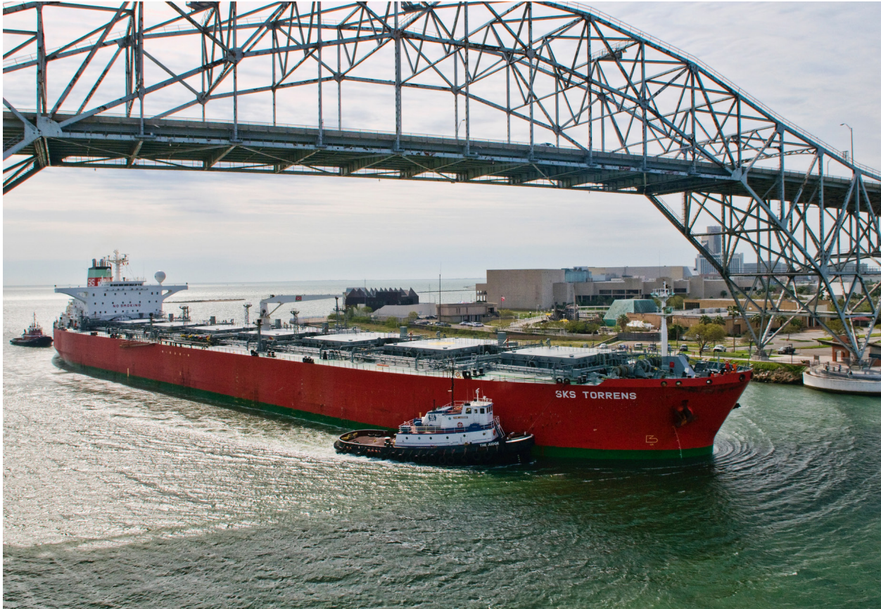
Photo courtesy of Port of Corpus Christi, Texas.
