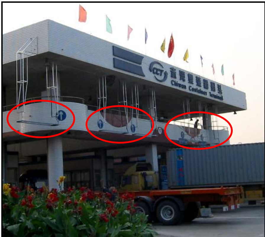
Chiwan Container Terminal (CCT) Shenzhen, China
