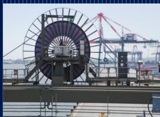
# 6 WATERSIDE / ON-DOCK INFRASTRUCTURE
