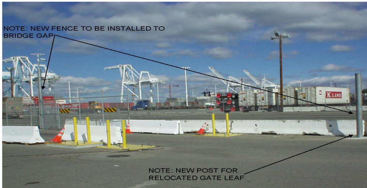
TBCT BERTH 25 – CHECKPOINT GATE LOOKING NORTHWESTERLY AT (E) DOUBLE LEAF SWII
