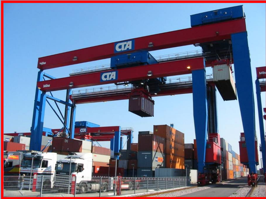
Container Terminal Altenwerder, Hamburg, Germany
