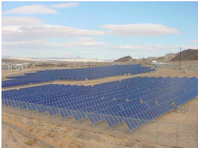
Photovoltaic Array MCAGCC 29 Palms, CA
