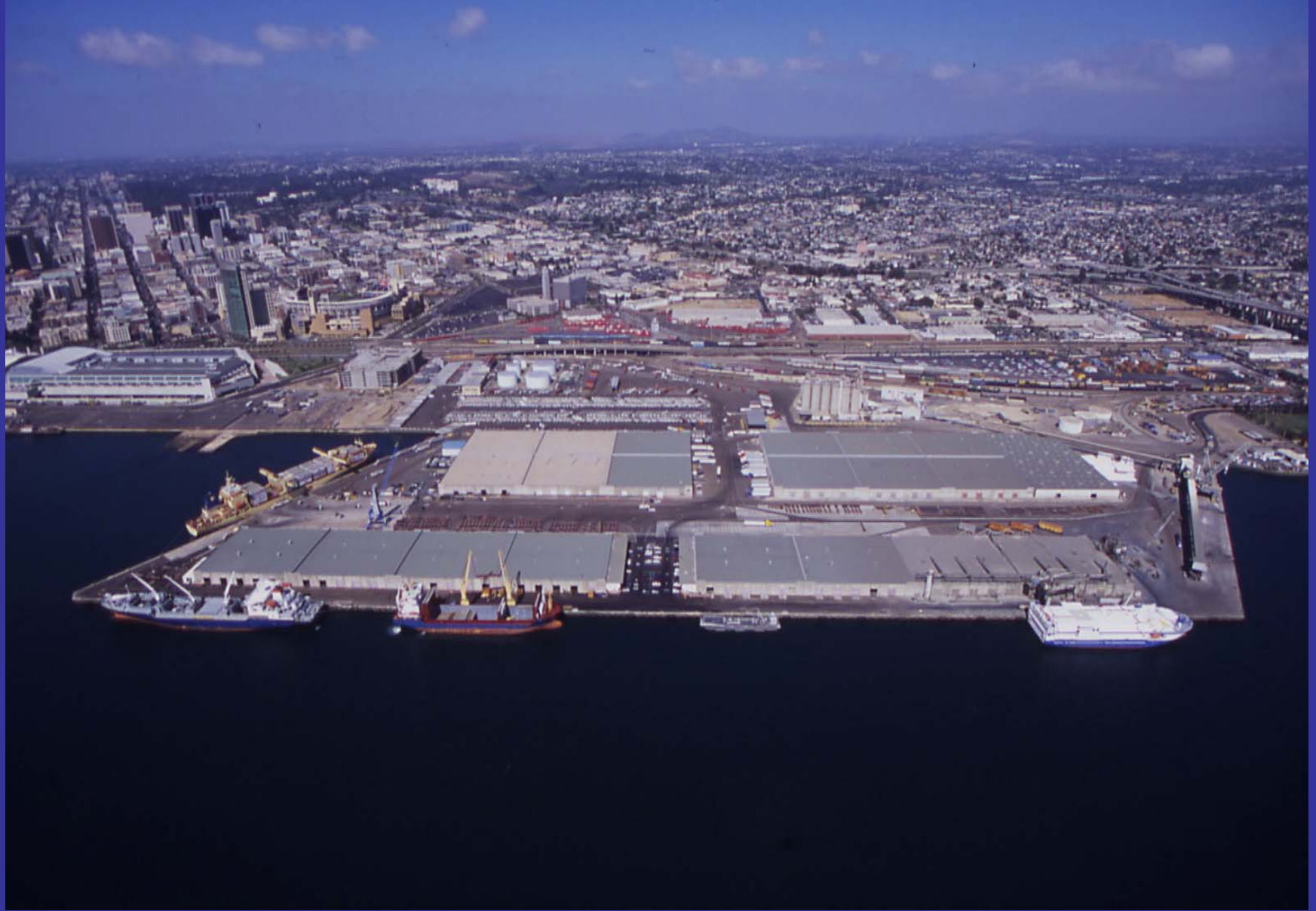
Tenth Avenue Marine Terminal
