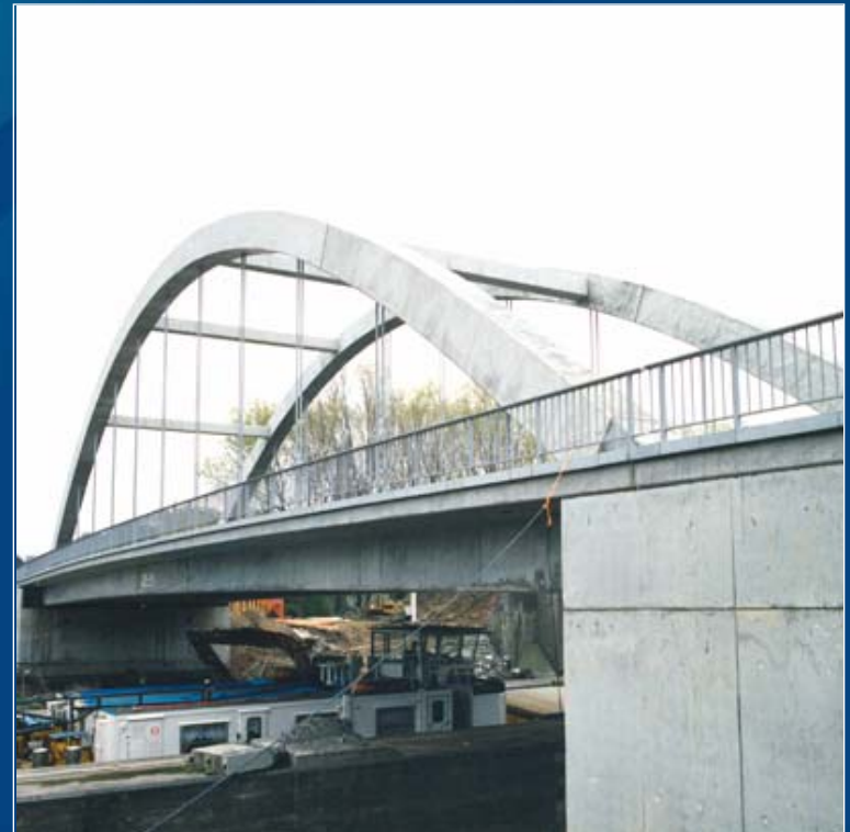
Bowstringbridge, removal of lock on the Upper Schelde
