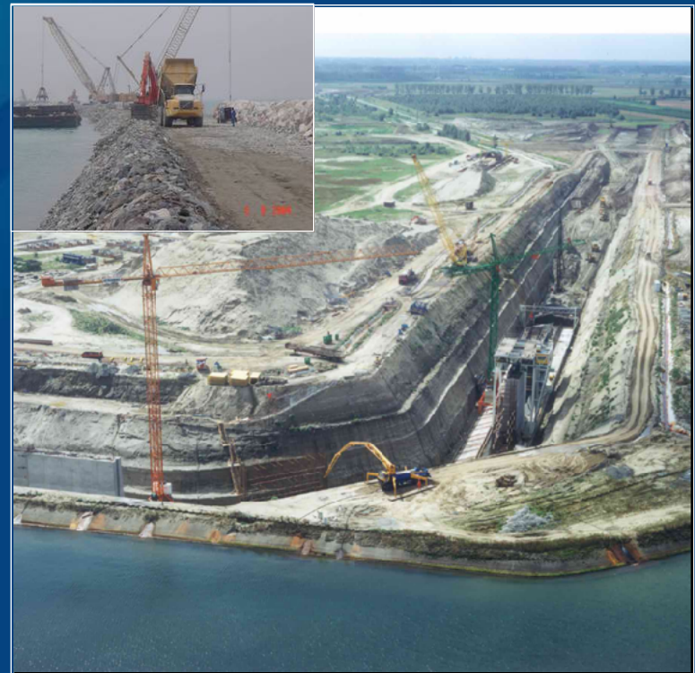
Quay wall construction at Verrebroek Antwerp - Belgium
