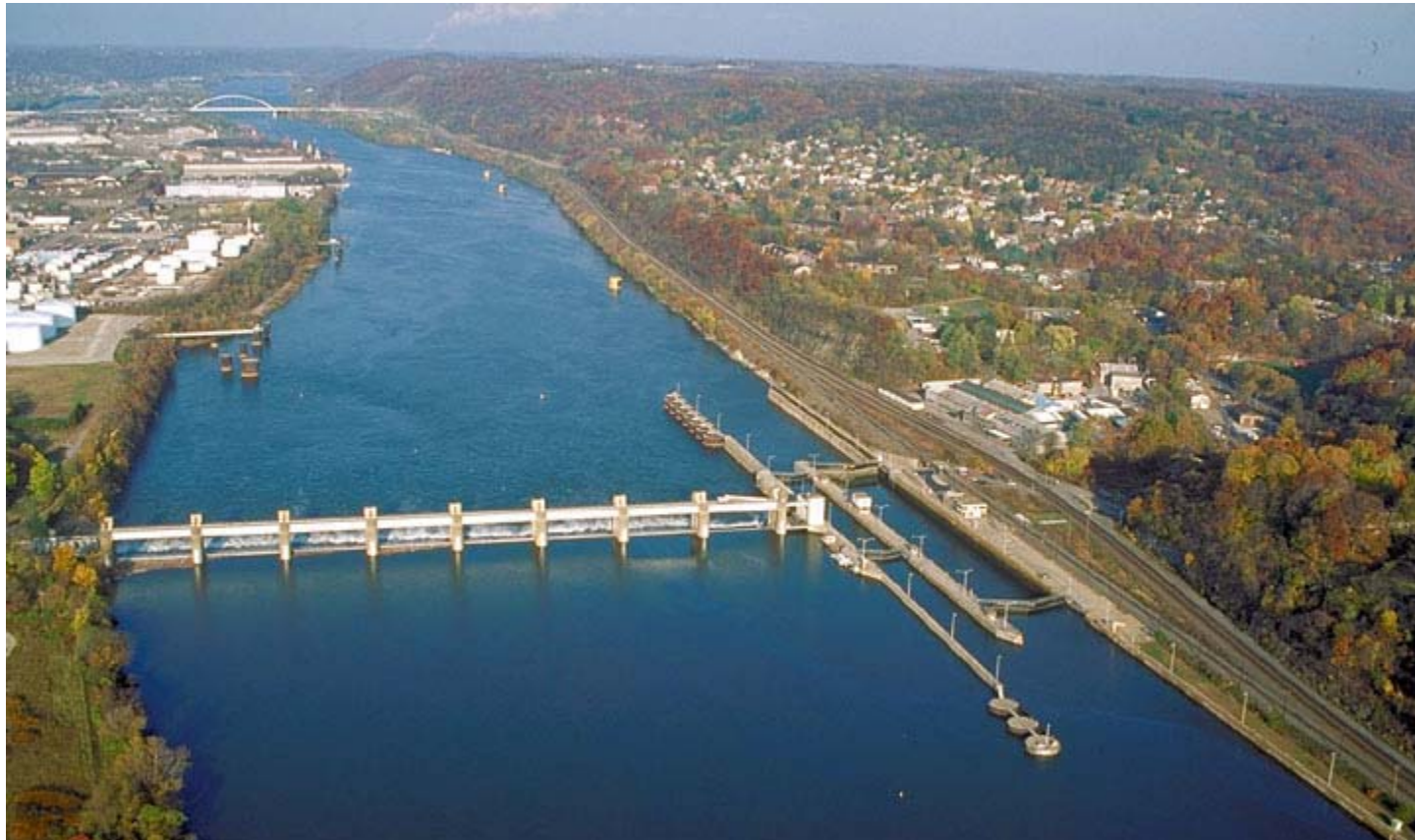
On the Ohio River downstream from Pittsburgh, Pennsylvania. Emsworth at Mile 6;
