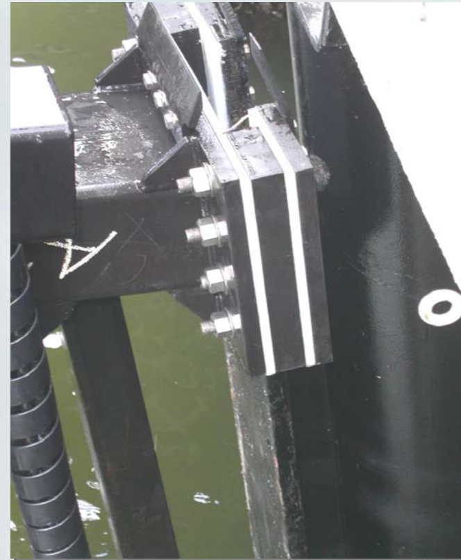
Guide shoe on H pile flange
