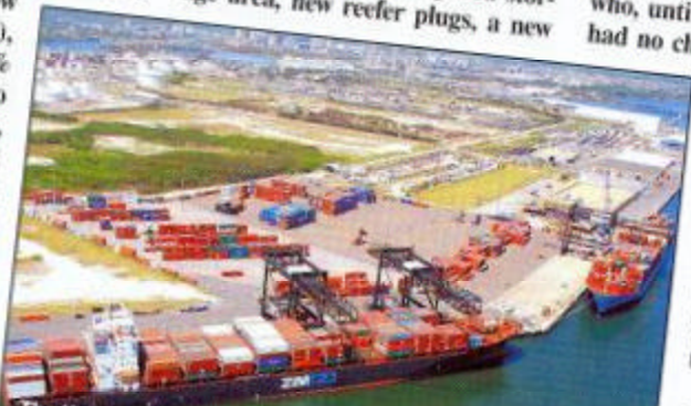
The Hooker's Point Container Terminal at the US port of Tampa
