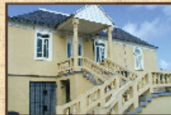
Entrance of Tharp House
