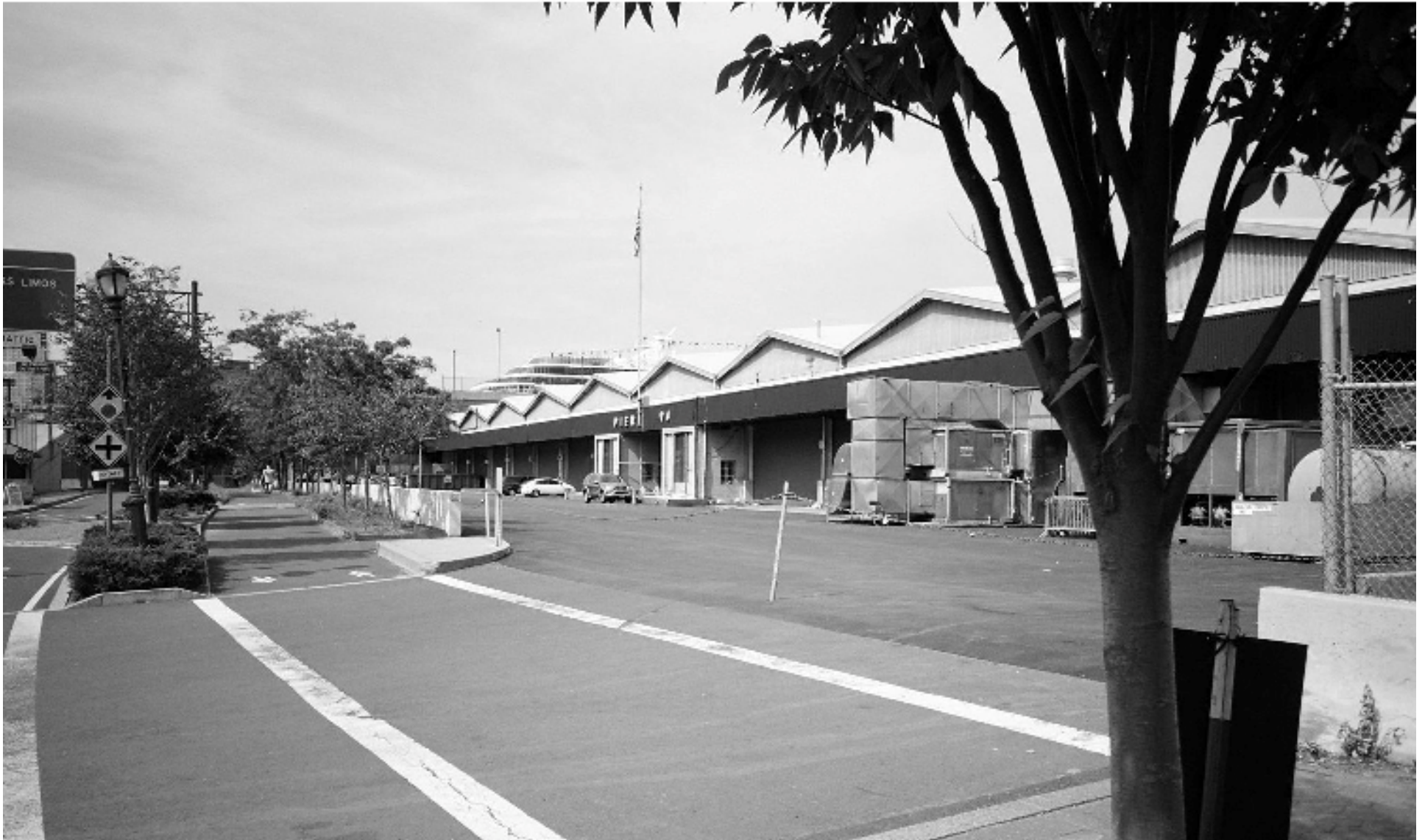
Piers 92/94 – Existing Main Entrance
