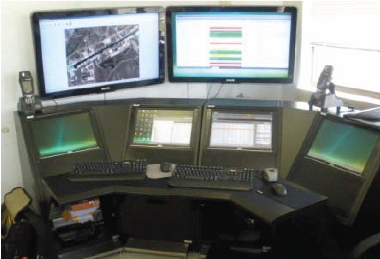
Security Office PACS Command Post
