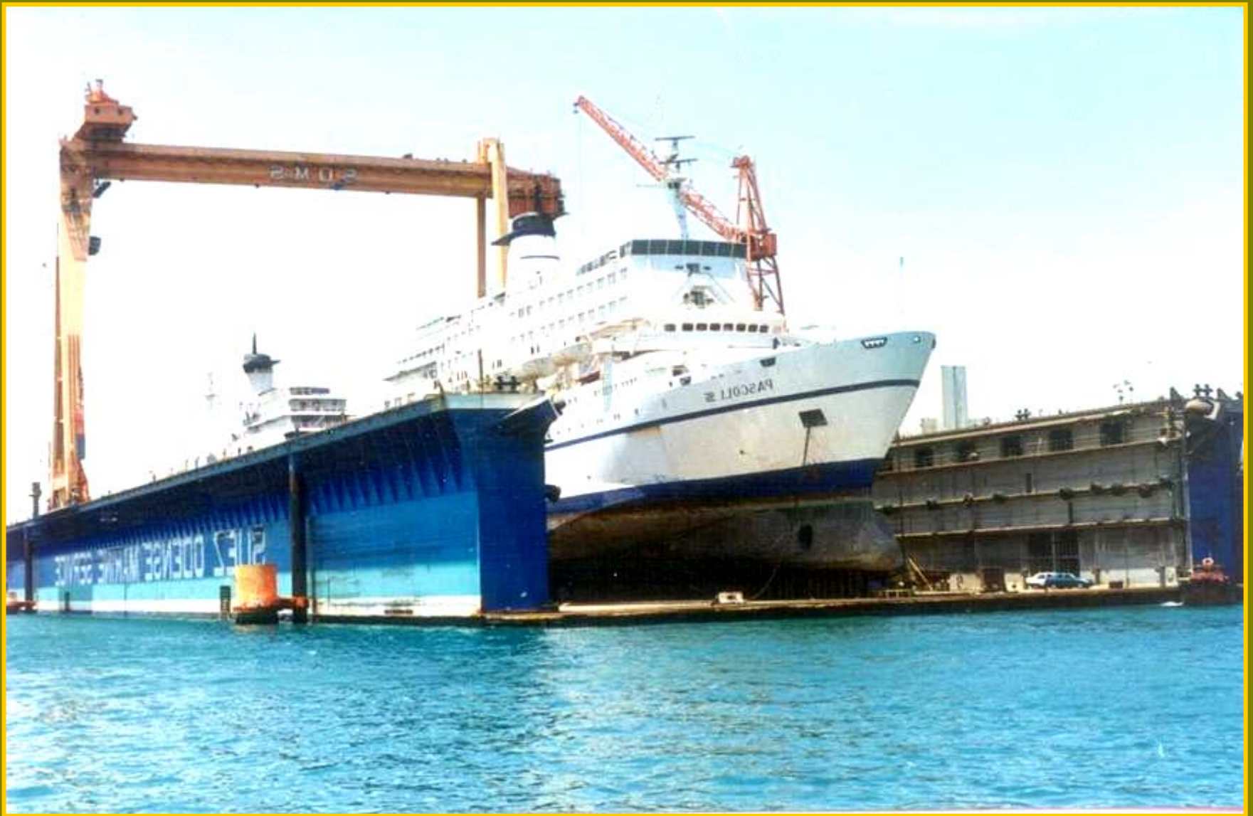
Floating dock of 55000 tons
