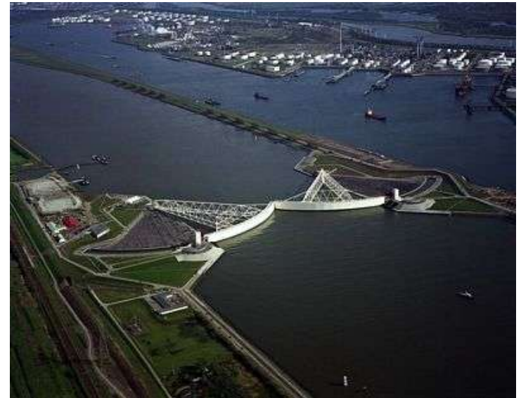
Deltaworks in the Netherlands
