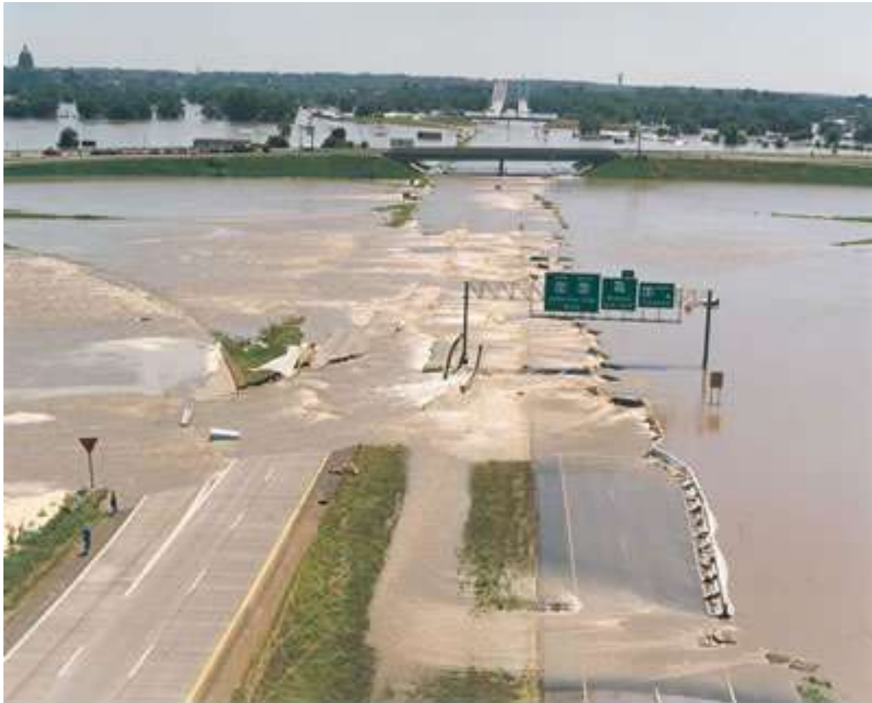
Aerial view of the Missouri River flooding on July 30, 1993, at U.S. Highway 54 just north of Jefferson City, Missouri, looking south (photography from the Missouri Highway and Transportation Department).
