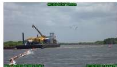
SCAT Field Photo - Boom Re
