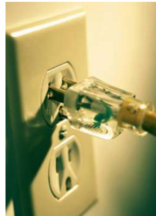
ANSI-NEMA 5-15R Wall Outlet and 5-15P Plug Type
