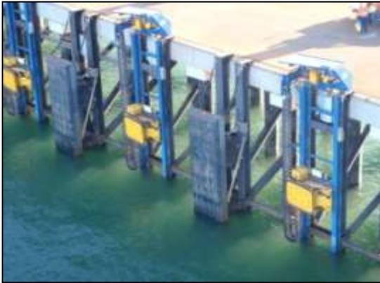
Vacuum pad installed on vertical rails
