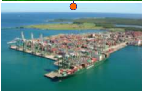
Colon Container Terminal
