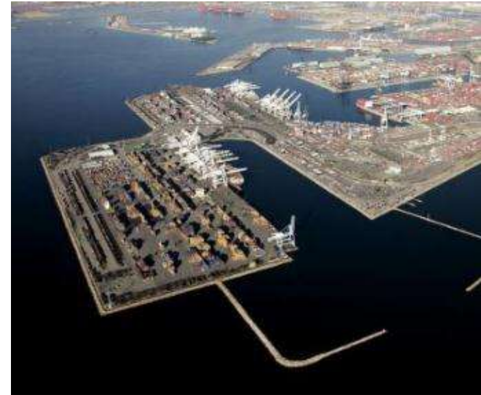
Pier J – Long Beach, CA
