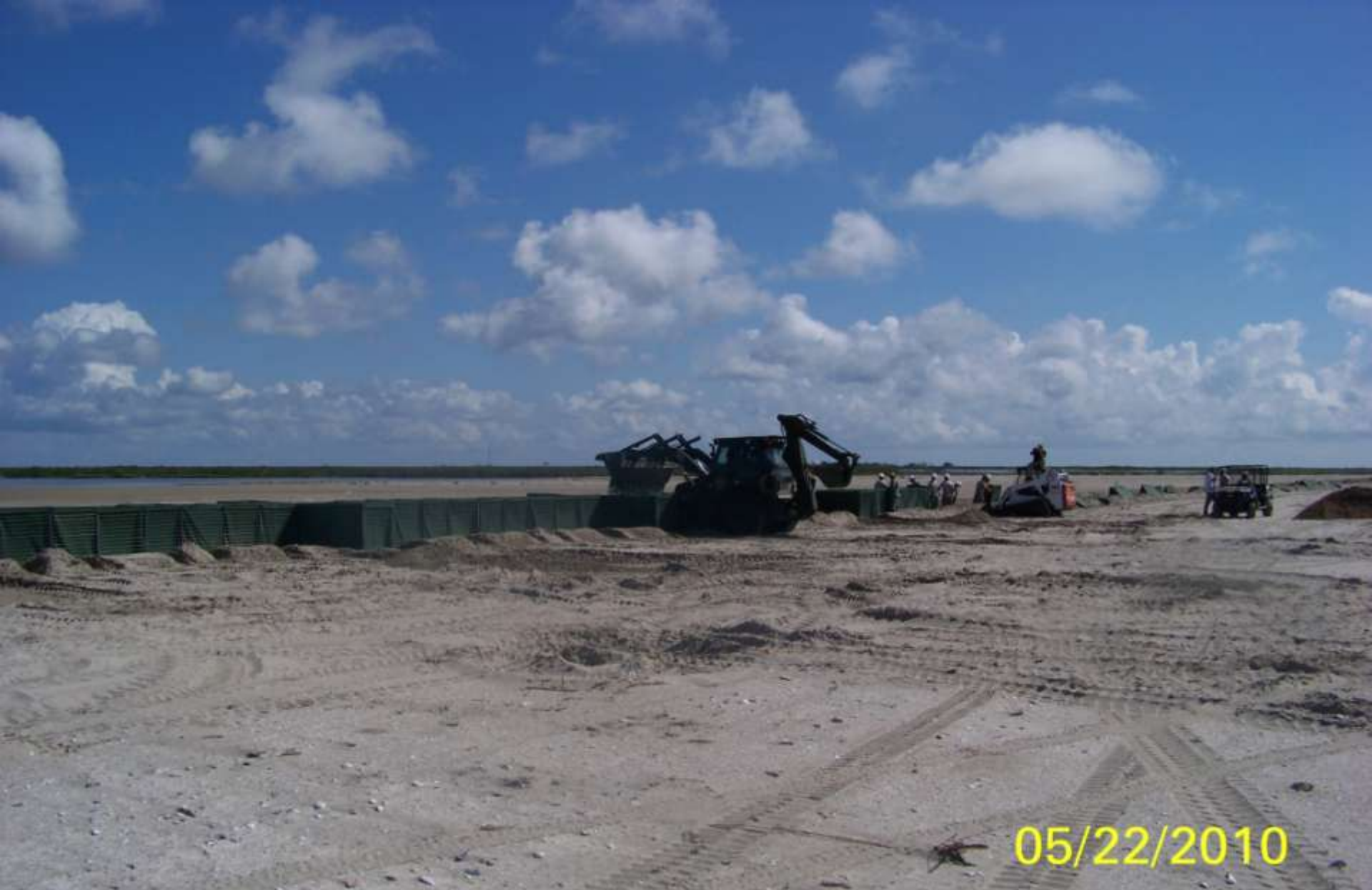
HESCO Baskets were installed to shore up beach dunes.
