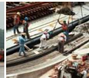
Tow track system
