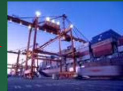
Container Terminal - Yantian, China
