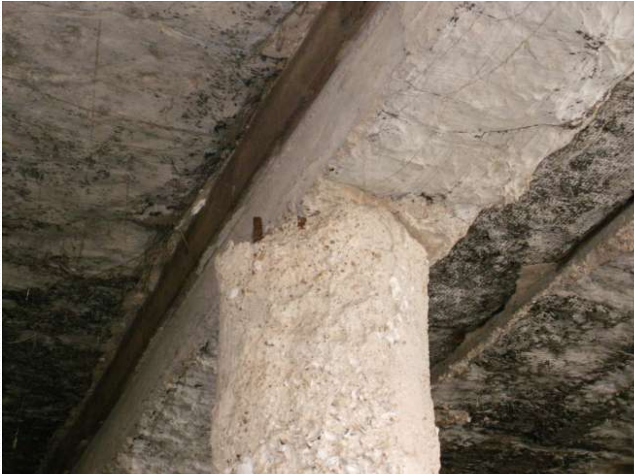
Column has partially shifted beneath beam.
