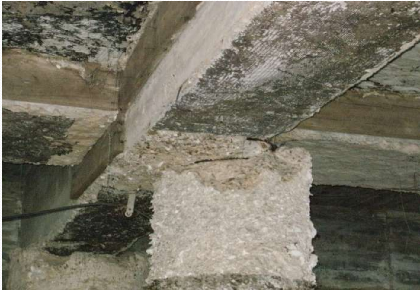
Column has shifted and broken free from overlying beam.
