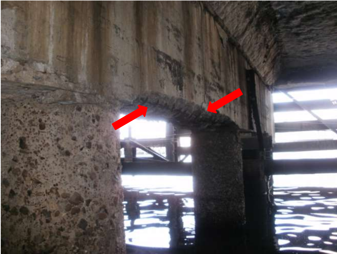
Corrosion to the Lower Reinforcement in the bottom of the beam.
