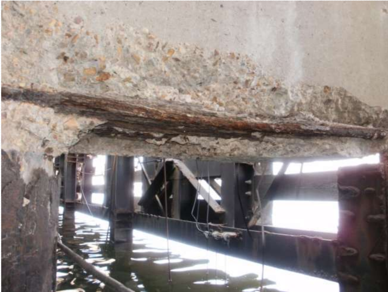
Exposed Reinforcement in the bottom of the beam.
