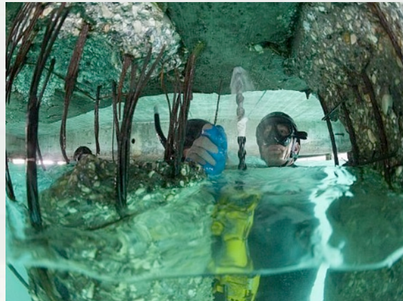
PORT-AU-PRINCE, Haiti (Feb. 6, 2010) Builder 2nd Class Andrej Paskevic, assigned to Underwater Construction Team (UCT) 1, drills guide holes into a damaged section of pier at the port in Port-au-Prince. (U.S. Navy photo by Mass Communication Specialist 2nd Class Chris Lussier/Released)
