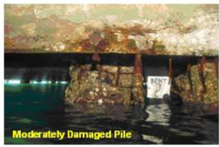
c) Examples of pile damage
