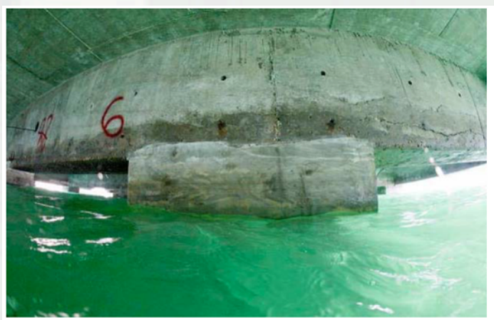
Figure 13 - Completed Formed Repair
