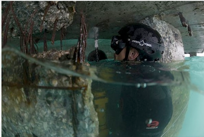
PORT-AU-PRINCE, Haiti (Feb. 6, 2010) Builder 2nd Class Andrej Paskevic, assigned to Underwater Construction Team (UCT) 1, drills guide holes into a damaged section of a pier. UCT-1 and Army Divers are conducting repair operations in the main seaport of Port-au-Prince. (U.S. Navy photo by Mass Communication Specialist 2nd Class Chris Lussier/Released)
