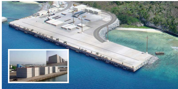
Kilo Wharf Extension
