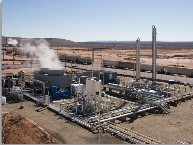
Clean Energy Boron Plant - Merchant Facility
