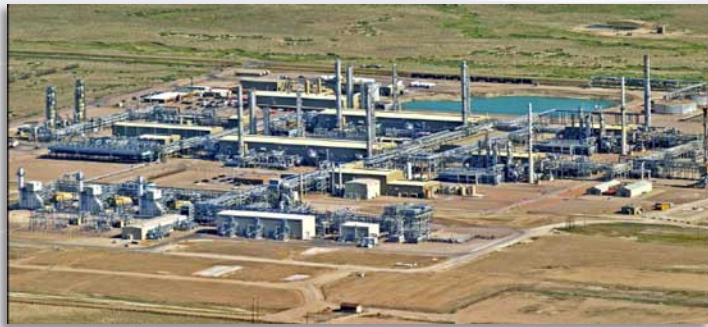
Exxon Shute Creek Gas Processing Plant
