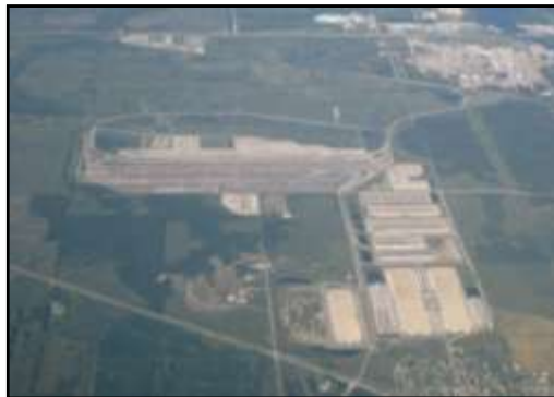
BNSF Logistics Park
