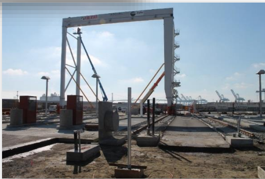
Civil Construction and Crane Equipment Integration
