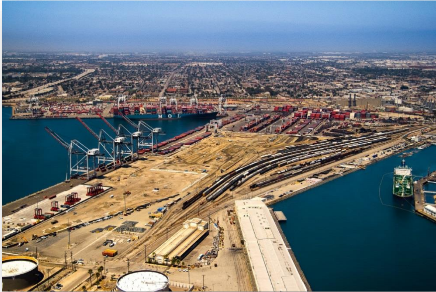
Project Site In Construction
