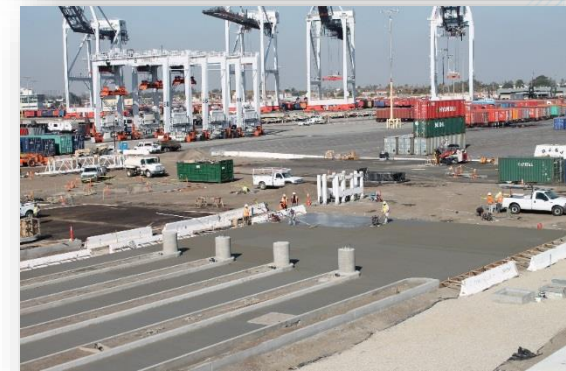
Berth 142-147 Active During Construction
