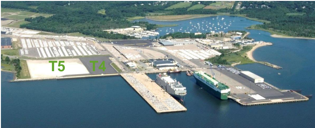
Terminal 4 and 5 project will add bulkhead cap, cleats, bollards, and fenders.
