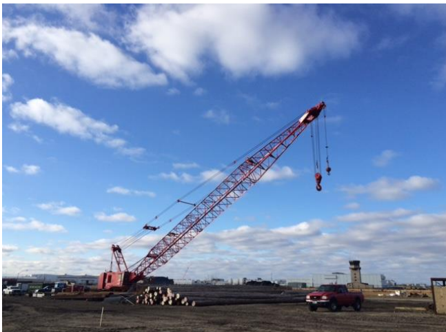
Crane on Quonset waterfront
